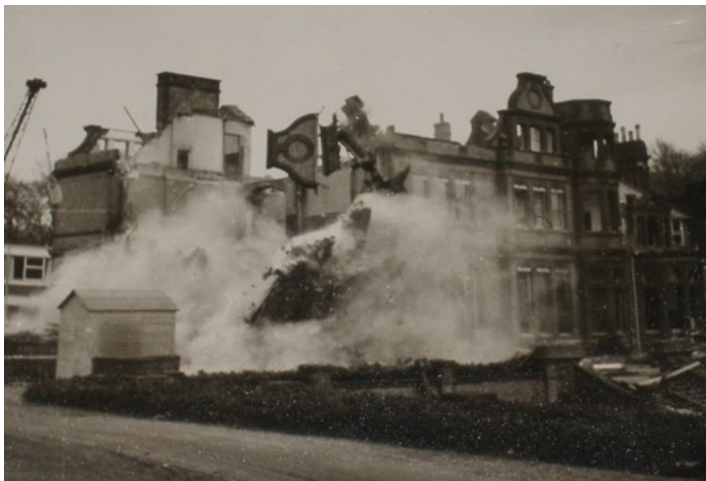
Ballards Mansion being knocked down in 1961.
